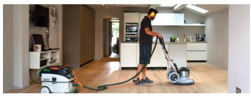
A buffer is used to give a silk-like texture to the floor before a wax oil or lacquer is applied
