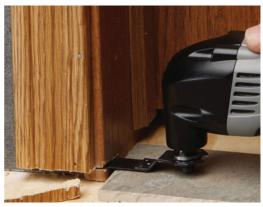
A really neat fit between the floor and the door jamb ... with the help of a special saw that enables ...
