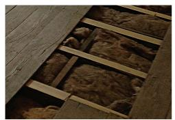
Fitting boards transversely to the joists
