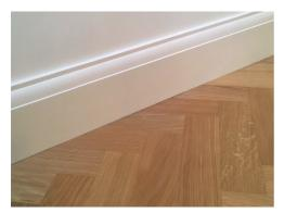
The skirting makes the perfect connection between the floor and the wall covering the necessary expansion gap between the two.
