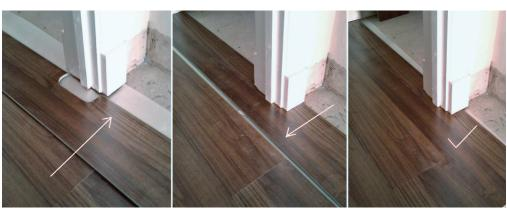
... the floor to slip underneath the door and the skirting
