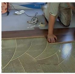
Gluing boards to a concrete screed
